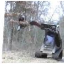
Vertical cutting along access road
